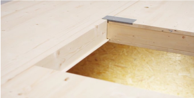
Large framing with trimmer and steel plates
