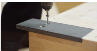
Large framing with trimmer and steel plates
