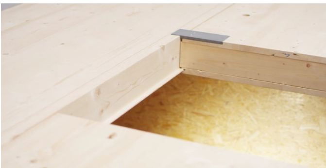
Large framing with trimmer and steel plates
