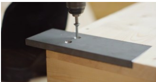
Large framing with trimmer and steel plates
