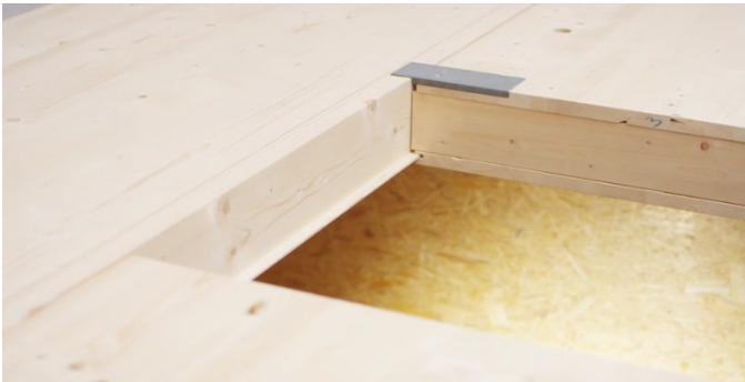
Large framing with trimmer and steel plates
